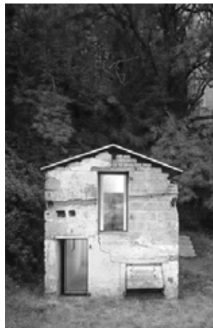
'Hous within a house'. 200-year-old abandoned pigsty in Rheinland-Pfalz, Germany, FNP Architekten, 2004
